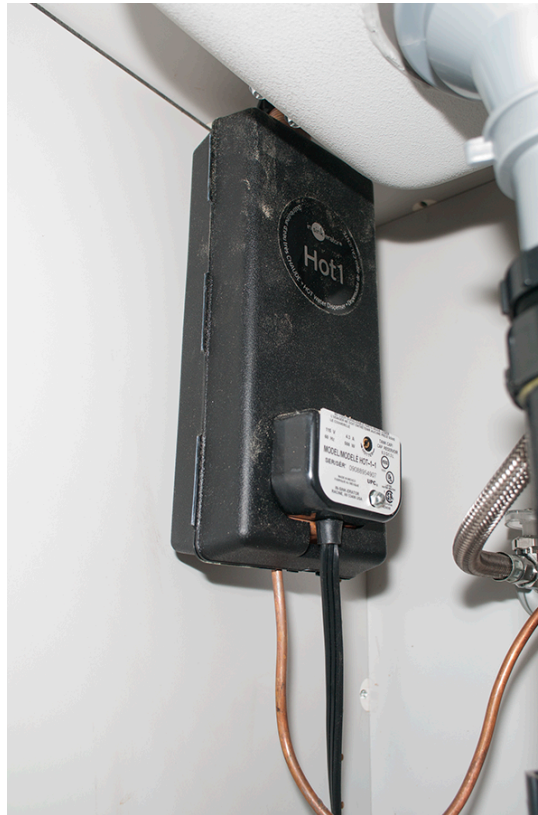
Figure 10 Small point-of-use, on-demand, electric water heater. (Skilled Trades BC, 2021) Used with permission.
