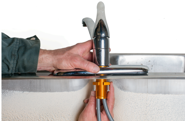
Figure 32 Installing a single-handle kitchen faucet. (Skilled Trades BC, 2021) Used with permission.
