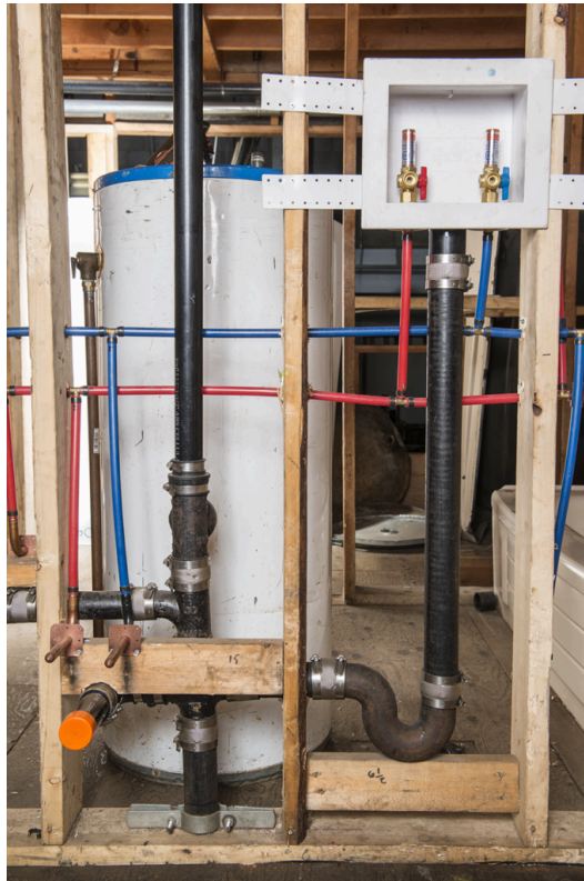
Figure 6 Laundry box for clothes washer and laundry tub. (Skilled Trades BC, 2021) Used with permission.
