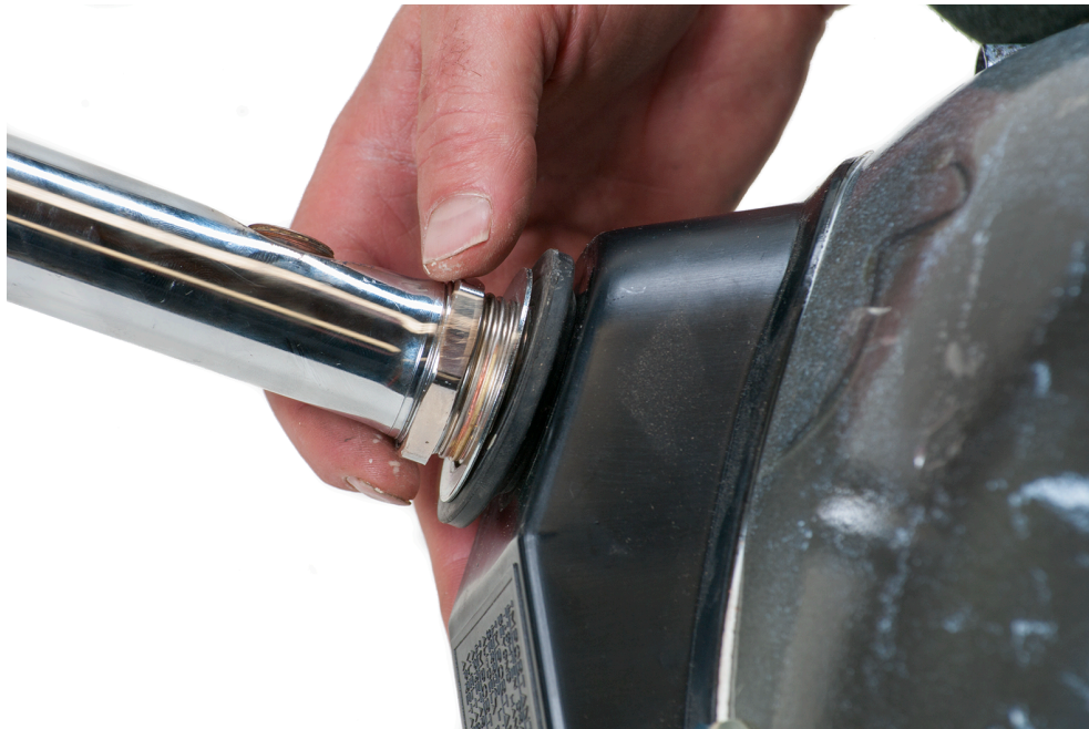
Figure 17 Install lower gasket, washer and locknut. (Skilled Trades BC, 2021) Used with permission.
