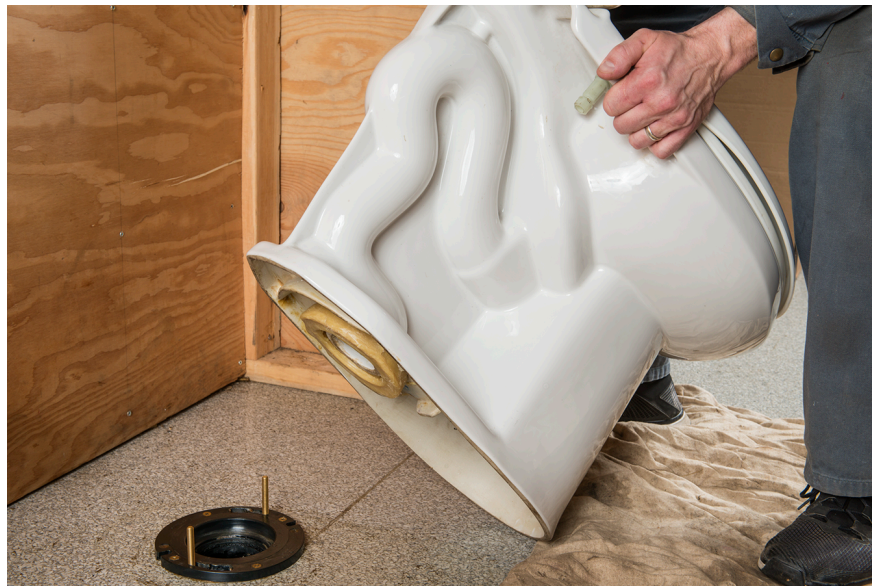
Figure 28 Placing toilet. (Skilled Trades BC, 2021) Used with permission.
