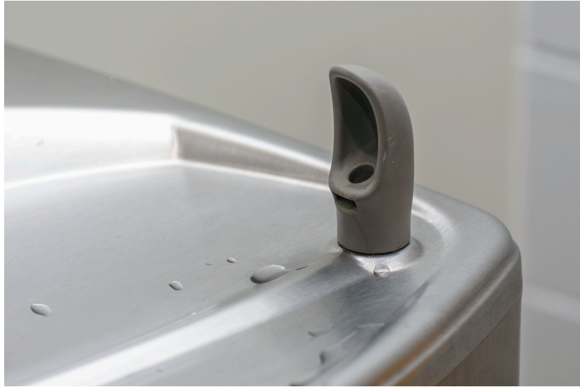
Figure 74 Drinking fountain bubbler. (Skilled Trades BC, 2021) Used with permission.
