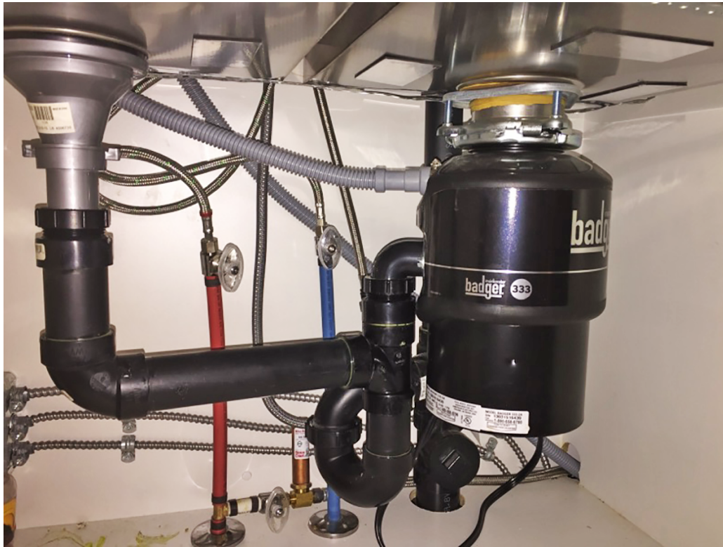
Figure 1 Garbage disposal installation. (Skilled Trades BC, 2021) Used with permission.
