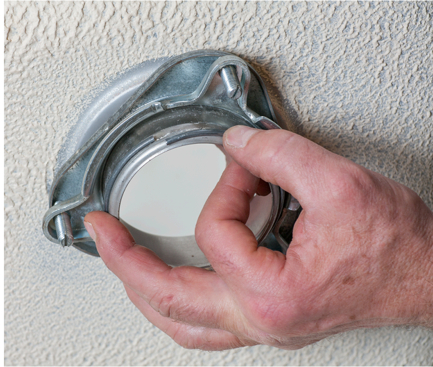
Figure 2 Standard flange drain body without threads. (Skilled Trades BC, 2021) Used with permission.
