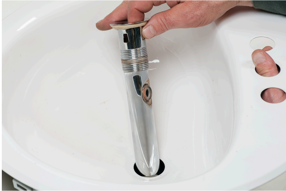
Figure 16 Insert drain plug fitting. (Skilled Trades BC, 2021) Used with permission.
