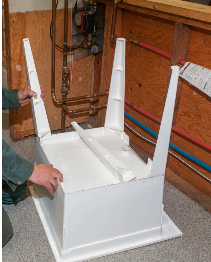
Figure 34 Installing a laundry tub. (Skilled Trades BC, 2021) Used with permission.
