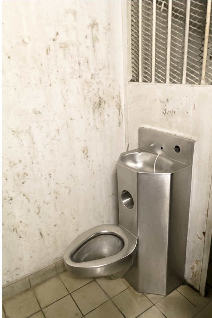
Figure 47 Stainless steel one-piece prison washroom unit. (Édouard Hue/Wikimedia Commons) CC BY-SA 3.0 ( https://creativecommons.org/licenses/by-sa/3.0/deed.en )
