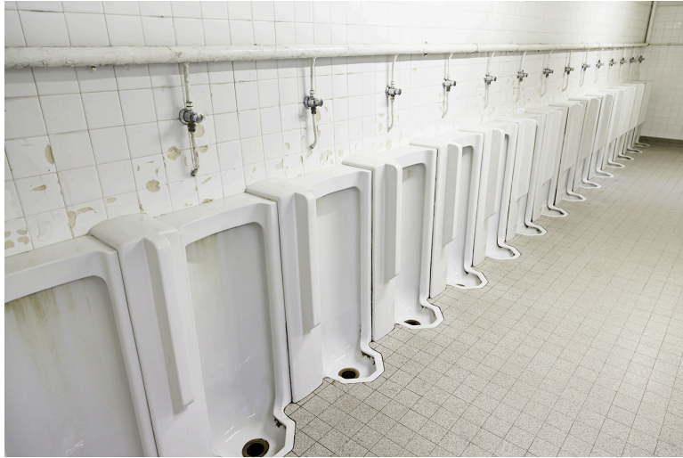
Figure 19 Stall urinal. (Skilled Trades BC, 2021) Used with permission.
