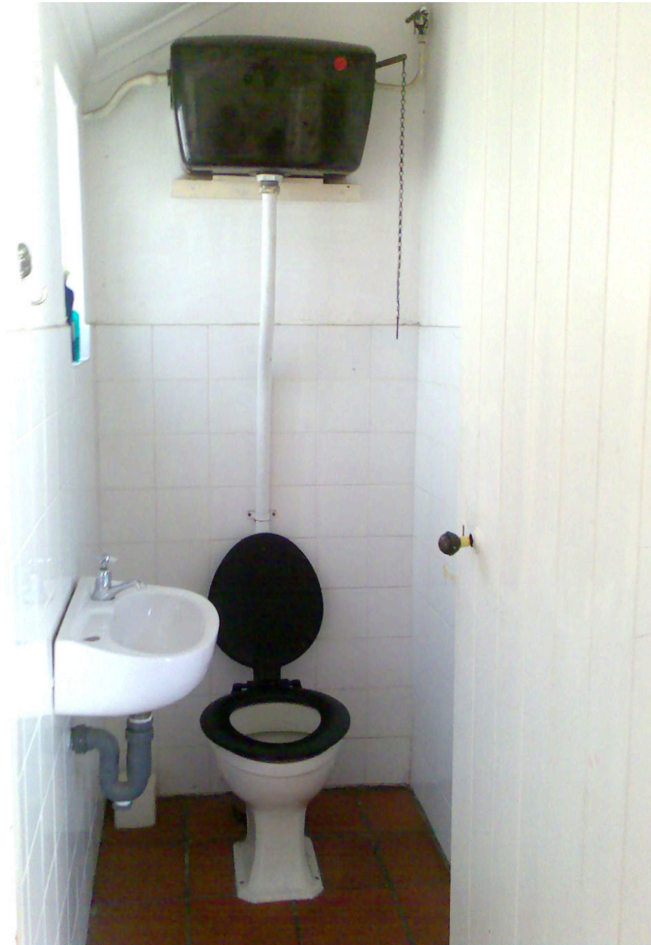
Figure 9 Floor-mounted, bottom outlet, high tank water closet. (Gregorydavid ( https://en.wikipedia.org/wiki/User:Gregorydavid ) at English Wikipedia) ( https://en.wikipedia.org/wiki/ ) CC BY-SA 3.0 ( https://creativecommons.org/licenses/by-sa/3.0/deed.en )
