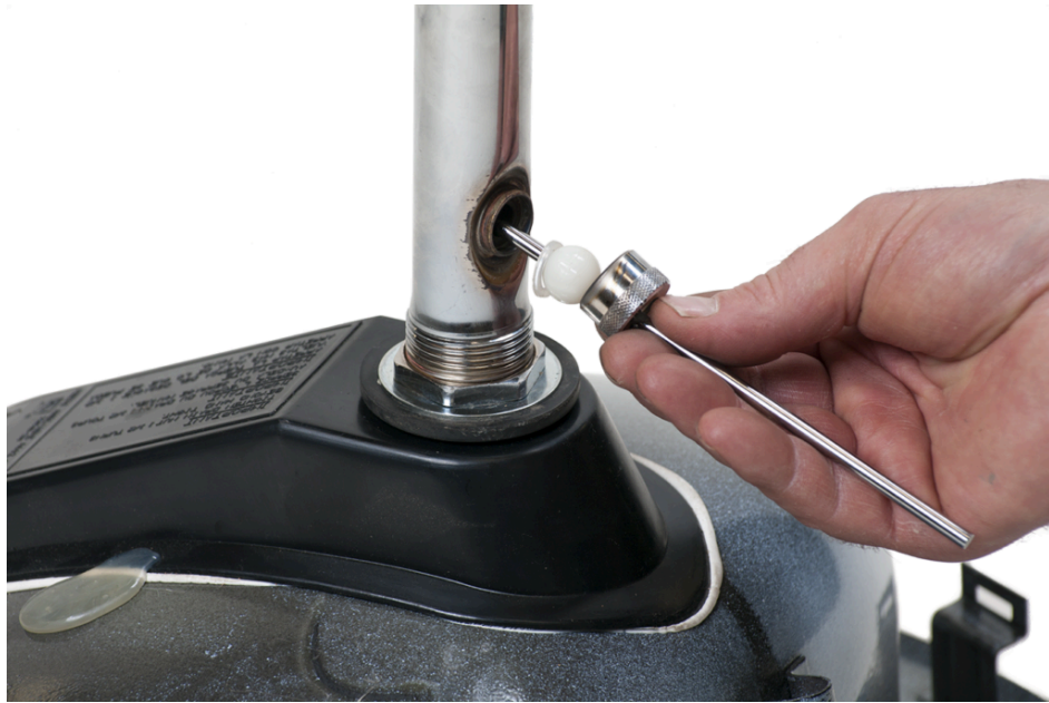
Figure 18 Install pivot rod. (Skilled Trades BC, 2021) Used with permission.
