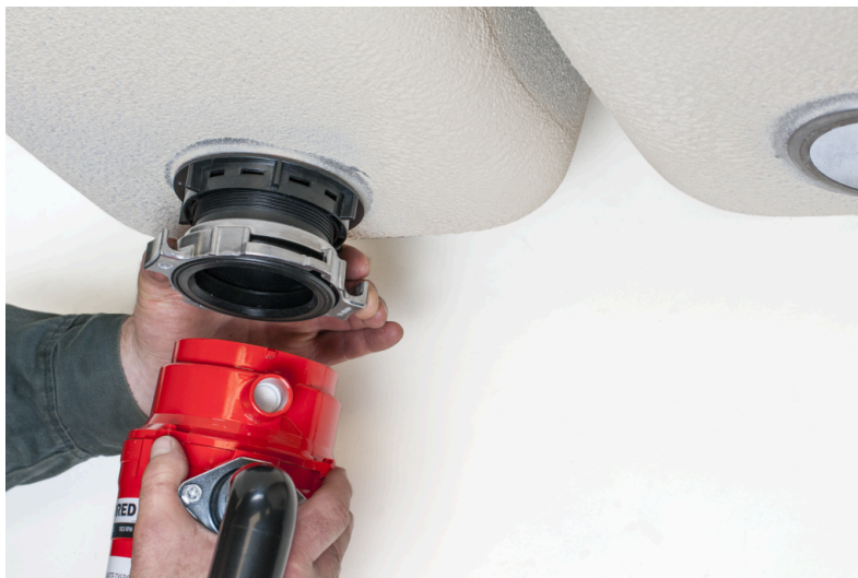
Figure 4 Mounting the garburator to the outlet fitting. (Skilled Trades BC, 2021) Used with permission.
