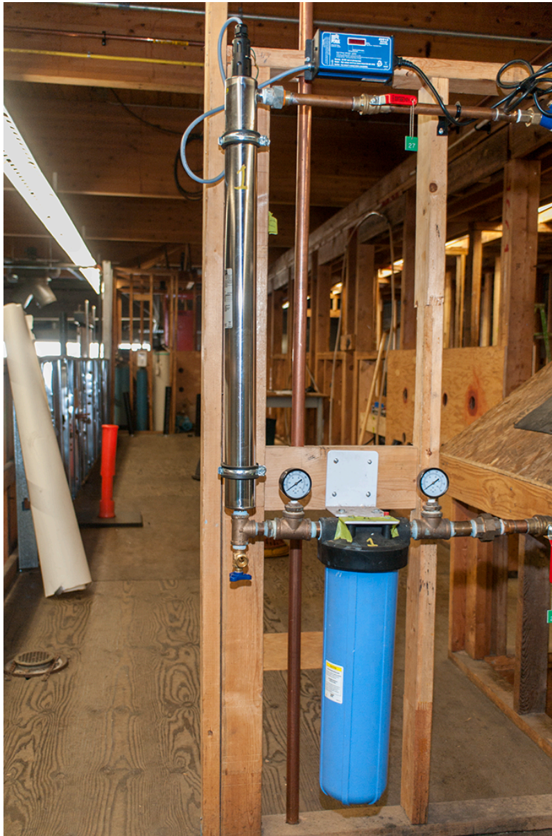
Figure 8 Ultraviolet water sterilizer with cartridge pre-filter. (Skilled Trades BC, 2021) Used with permission.
